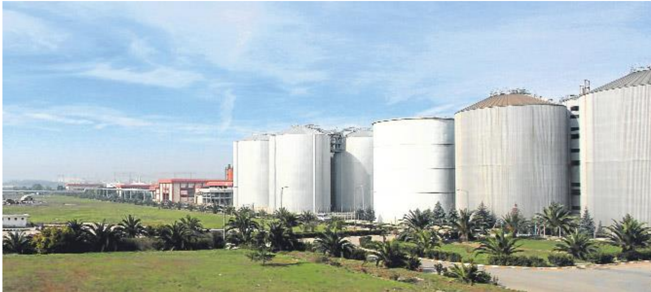
Istanbul-Tuzla Sludge Digesters
