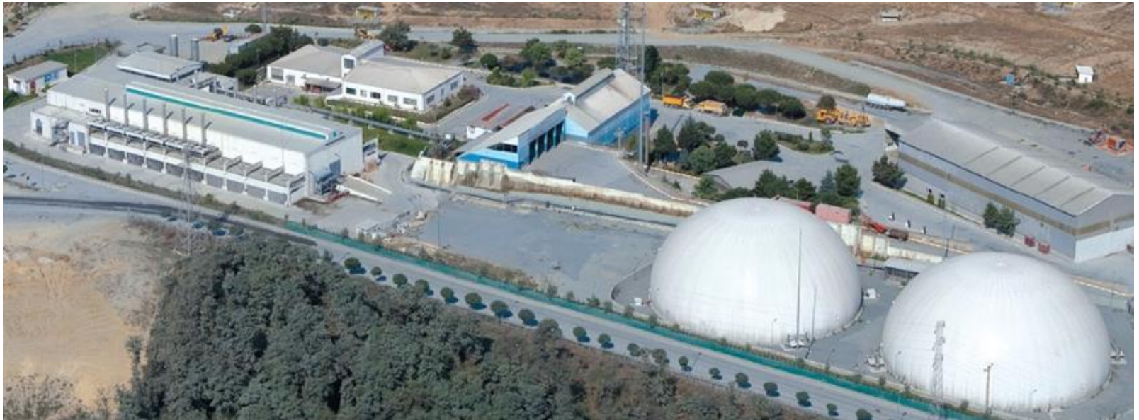
Istanbul Odayeri landfill gas to energy plant, 33.8 MW
