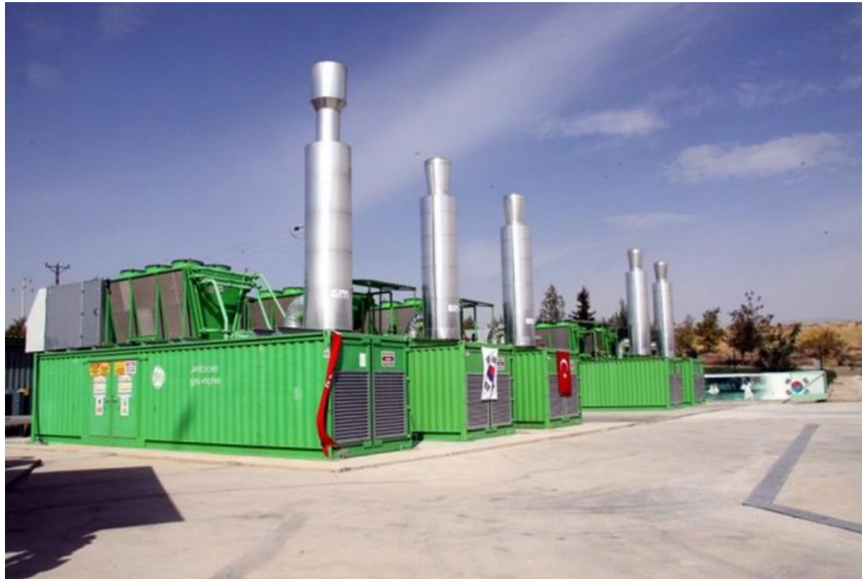
Gaziantep landfill gas to energy plant, 5.6 MW
