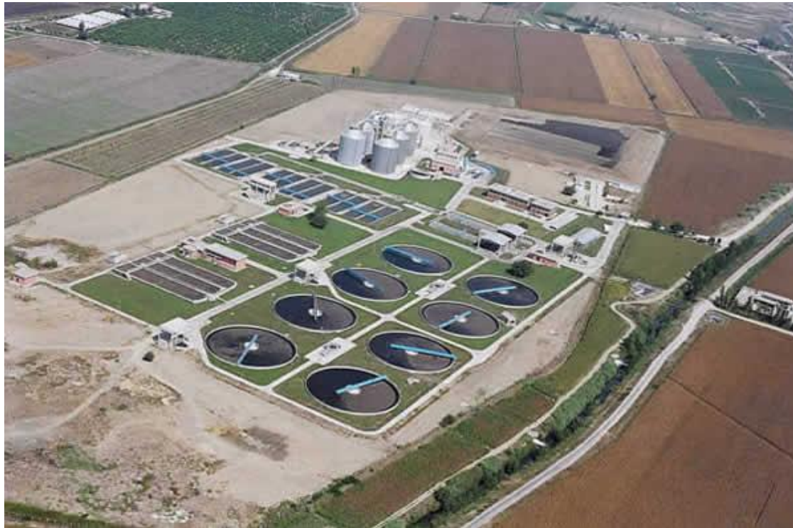
Adana Sludge Digesters
