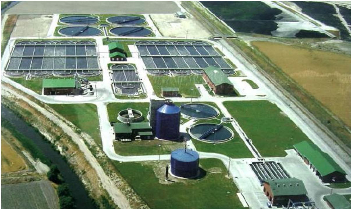
Kayseri Sludge Digester
