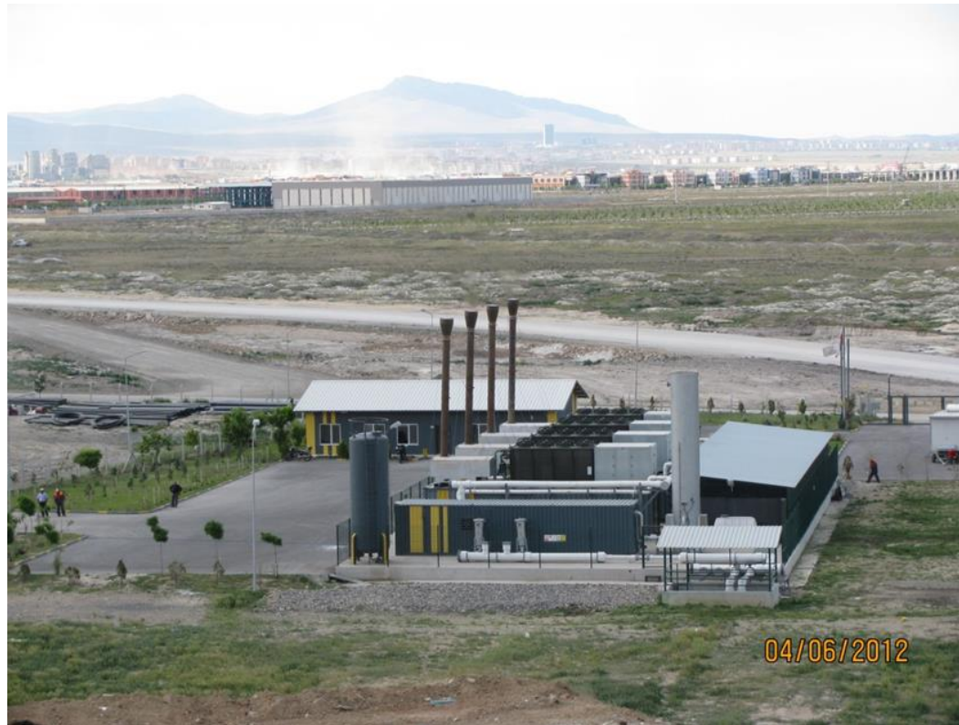
Konya landfill gas to energy plant, 5.7 MW
