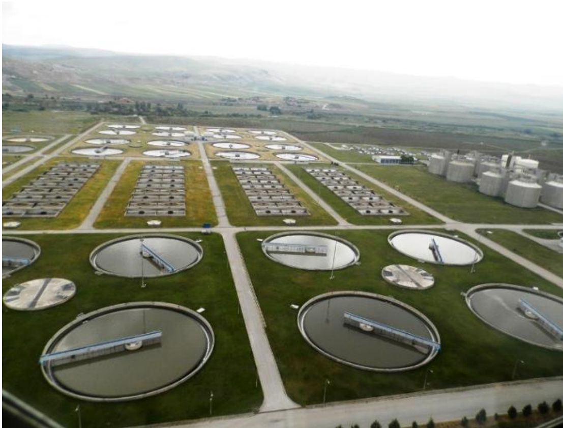
Ankara Sludge Digesters
