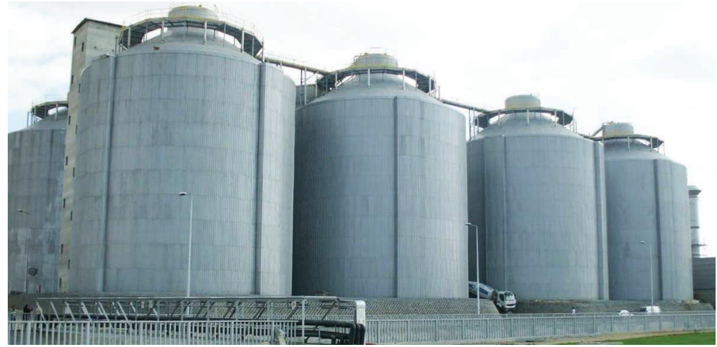
İstanbul-Ambarlı Sludge Digesters
