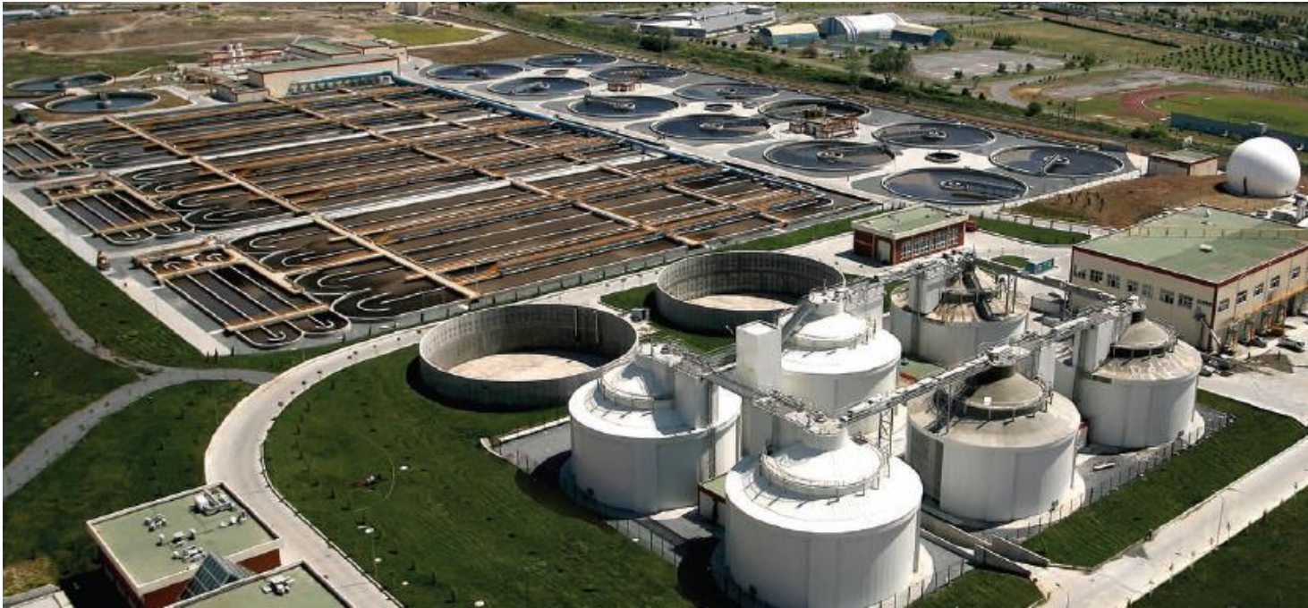
Istanbul-Ataköy Sludge Digesters
