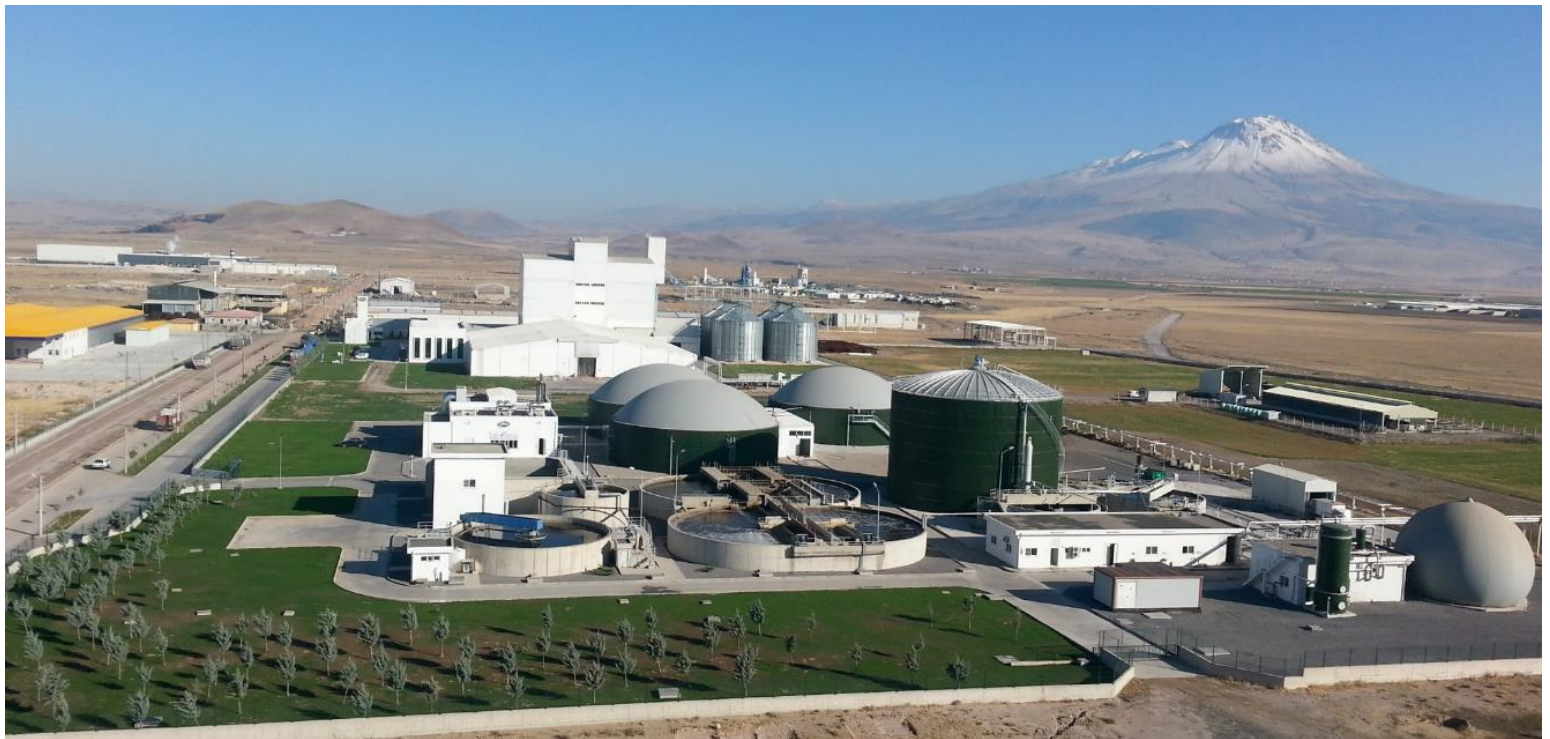
Sutas Aksaray Farm Digester
