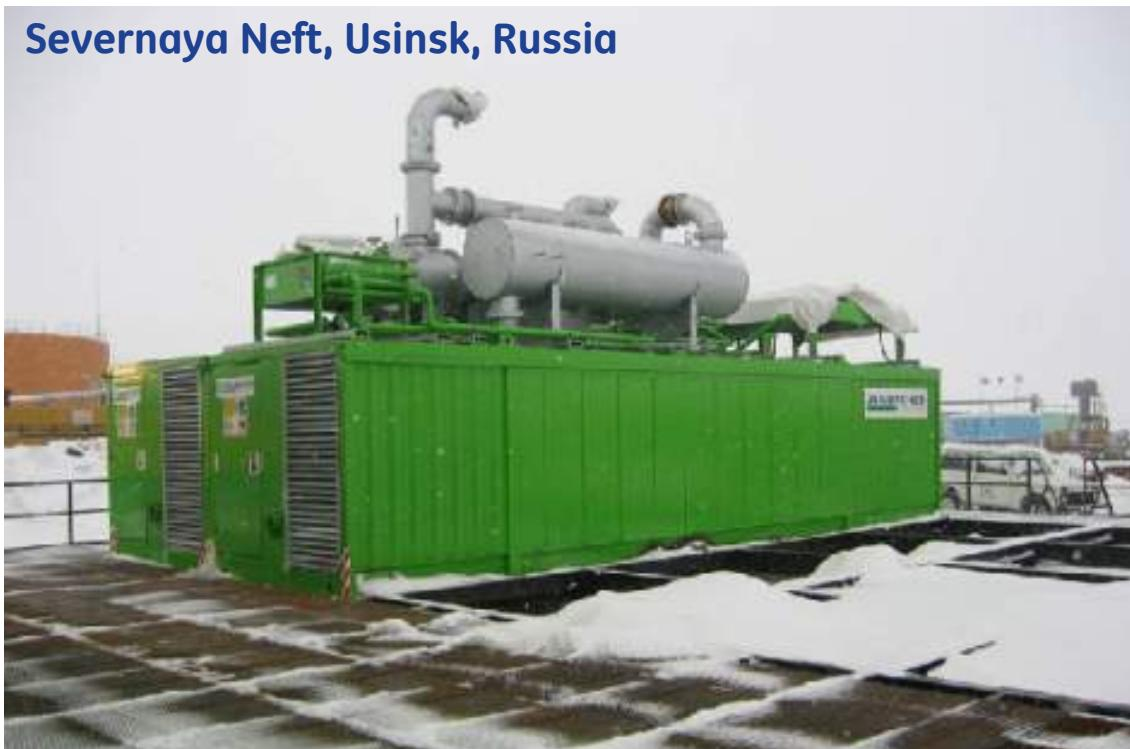
Provides heat & power using **associated gas** from the oil production site near the Arctic Circle ... avoids the need for **8M liters of diesel** annually
