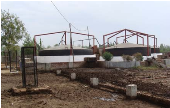
Biogas plants at Gaushala
