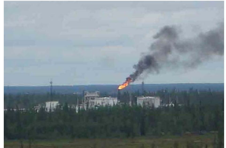
Booster pump station 升压泵站
