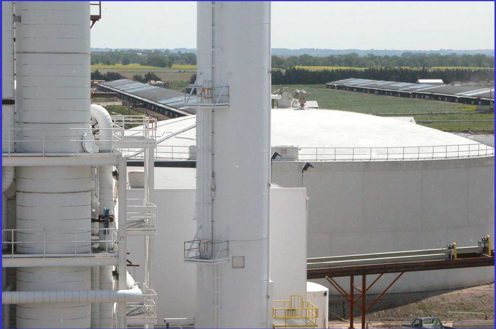
Pictured: Ethanol refinery towers (front), an anaerobic digester (center), and the feedlot (back).
