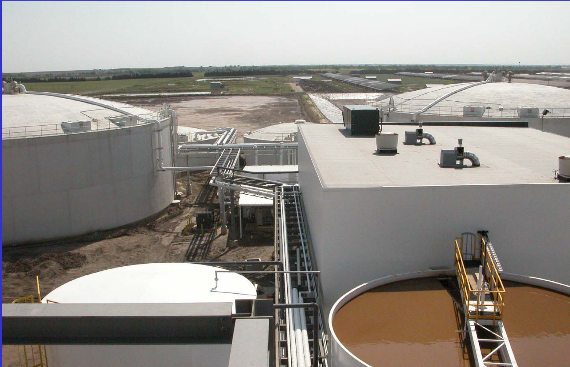
A view from the ethanol refinery of the anaerobic digesters, support systems, manure lagoon and feedlot.
