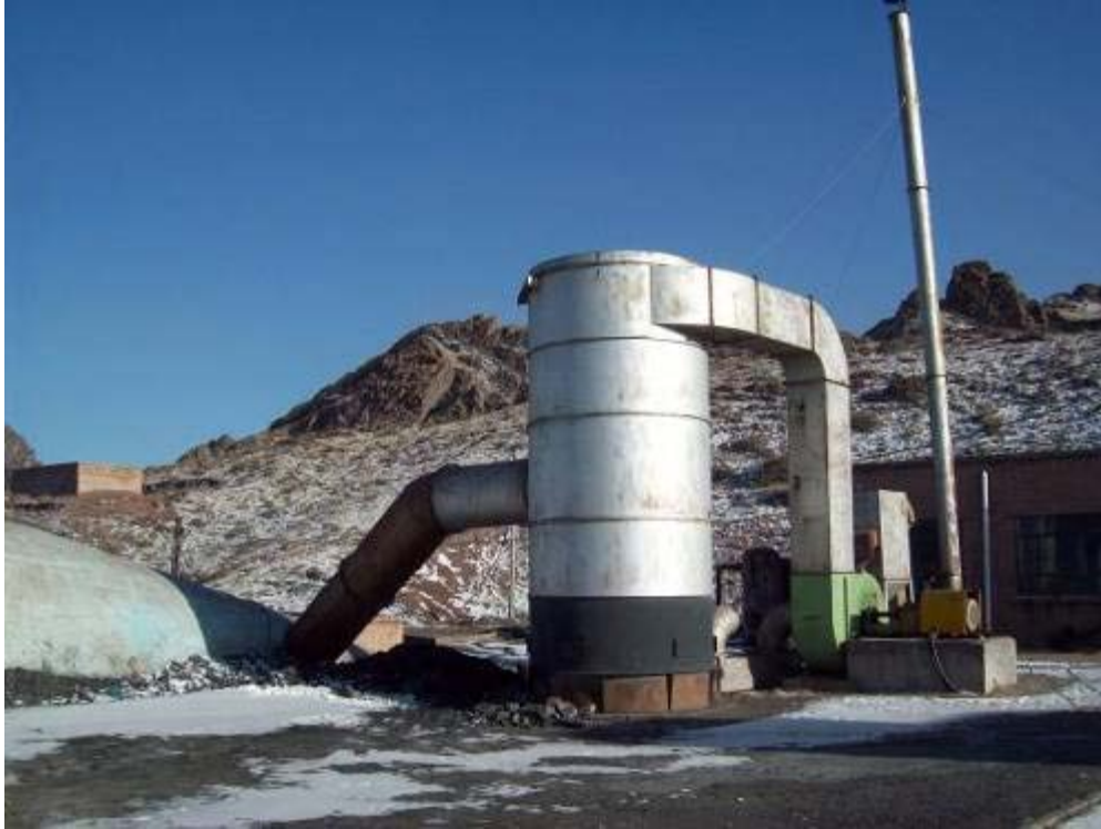
Figure 1.9: Example of Current Ventilation Drift Heating Arrangements
