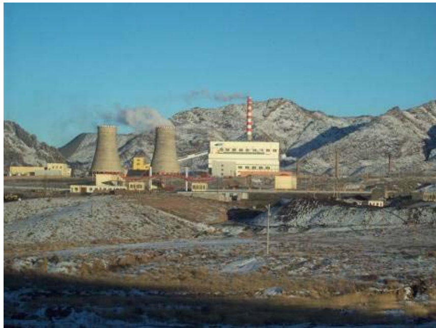
Figure 1.10: 18-MWe Thermal Power Plant for the Erdoaling Mining Area
