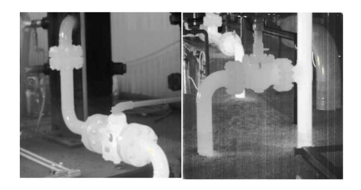
•Leaking bypass valve results in leakage from discharge to suction scrubber. 经过阀门的泄露引起了从排出到吸气口清洁器的泄露
