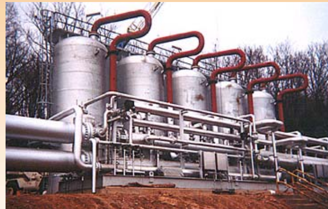
Desiccant Dehydrator Unit Source: GasTech
