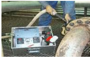
Oil & Gas Systems
