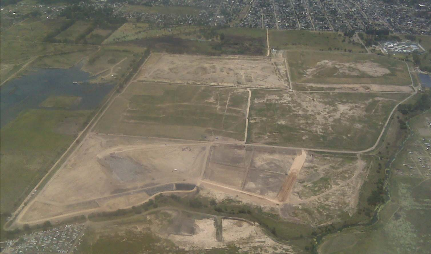
Aerial Photograph of González Catán Landfill
