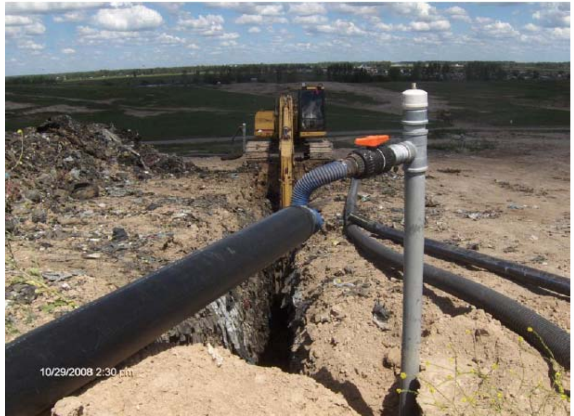
Installation of deep trenches
