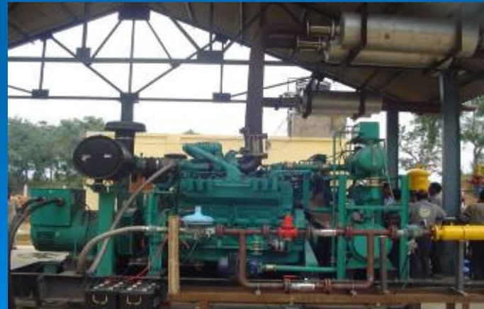
Gas Based Generator at Moonidih
