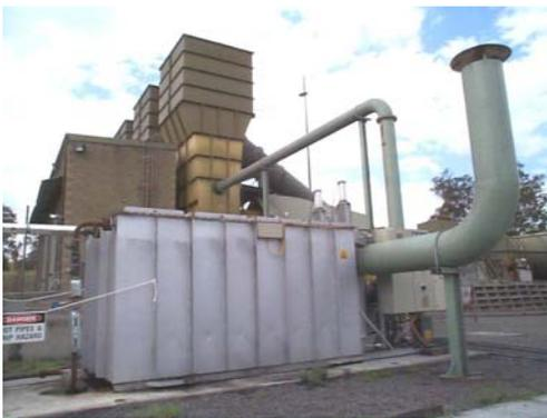
MEGTEC Thermal flow reversal reactor
