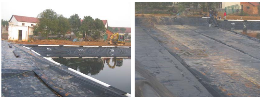
Cover installation at Haidong Ecological Agriculture Company
