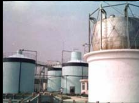
Project activity condition: Biogas digester with co- generation and aerobic treatment of liquid residue
