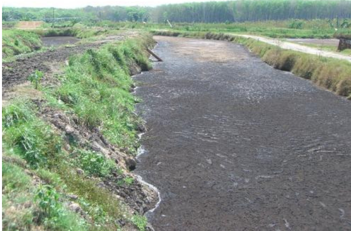
Figure 3-18: Conventional Anaerobic Lagoon
