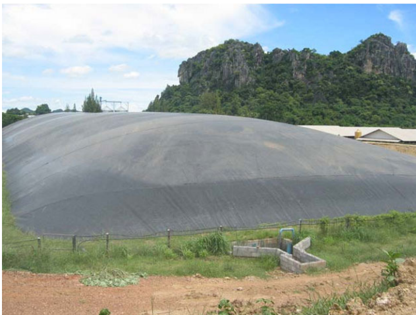
Figure 4-5: Covered Anaerobic Lagoon (CovAL) System
