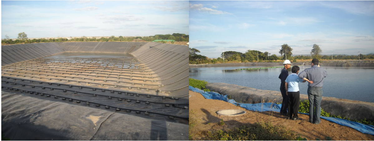
Figure 3-21: Covered Anaerobic Lagoons at Thai Roong Ruang Energy
