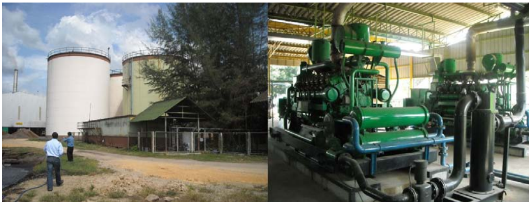
Figure 3-19: CSTR Biogas Technology and Biogas Power Generators in Asian Palm Oil
