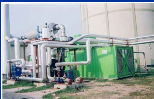
GAS ENGINE AND WASTE HEAT RECOVERY UNIT
