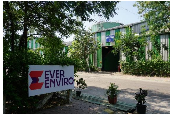
Figure 8: India's largest bio-CNG plant
