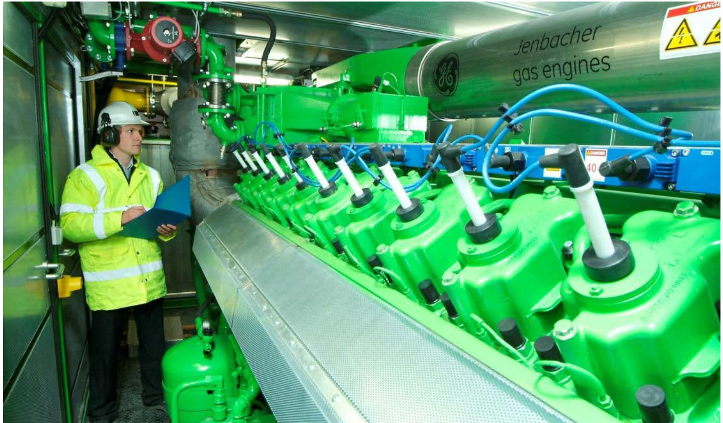
Failure to appreciate that gas engines need expert maintenance
