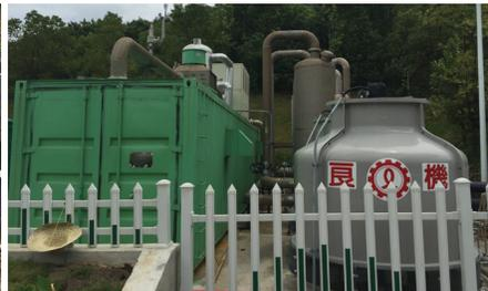
Biogas from landfill used to create pipeline quality natural gas (China)
