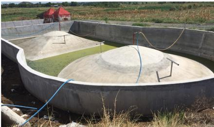
Biogas from animal waste anaerobic digester used as cooking fuel (Philippines)
