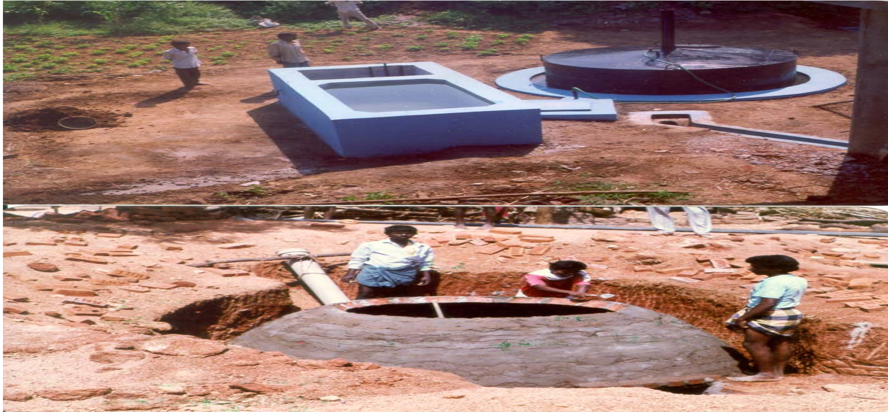
Biogas Plant Designs Top: Floating drum Bottom: Fixed dome
