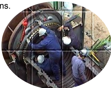
Dry seal installation
