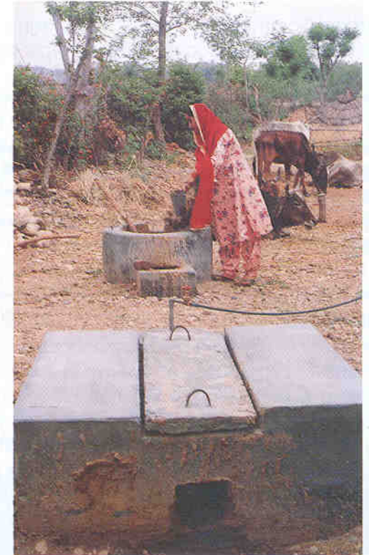
A Deenbandhu Biogas Plant at Deoli Village, Himachal Pradesh.
