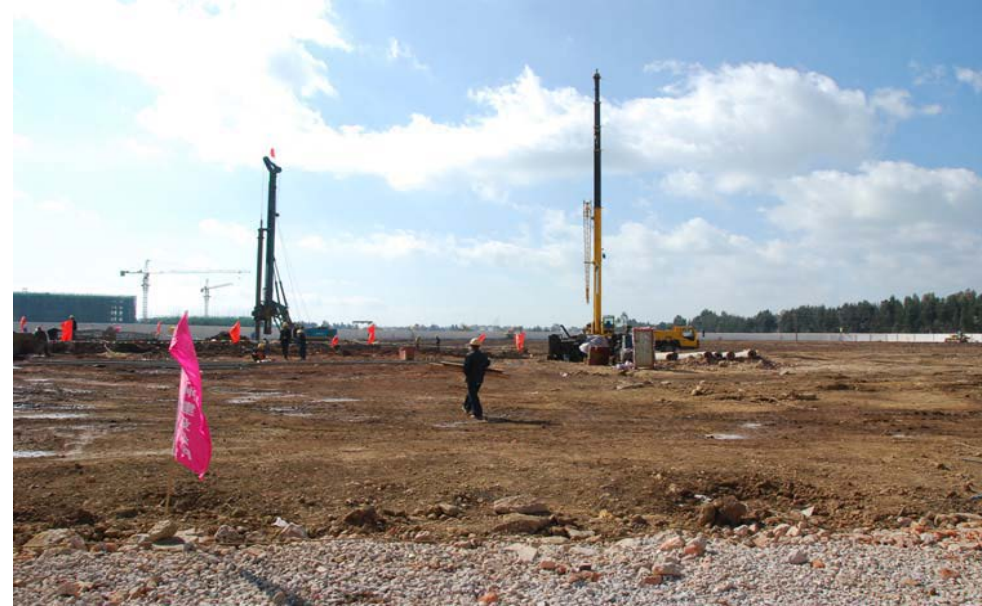
Project Site in Kunming City
