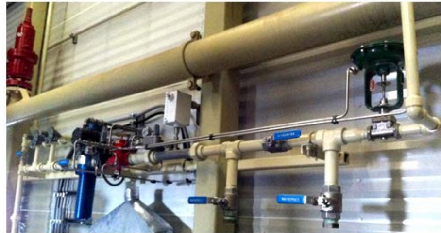
SlipStream® valve train redirects previously vented gas into engine's air intake as fuel
