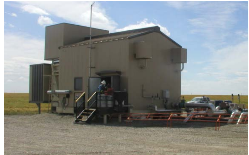
Typical compressor building in the Clearwater Business Unit
