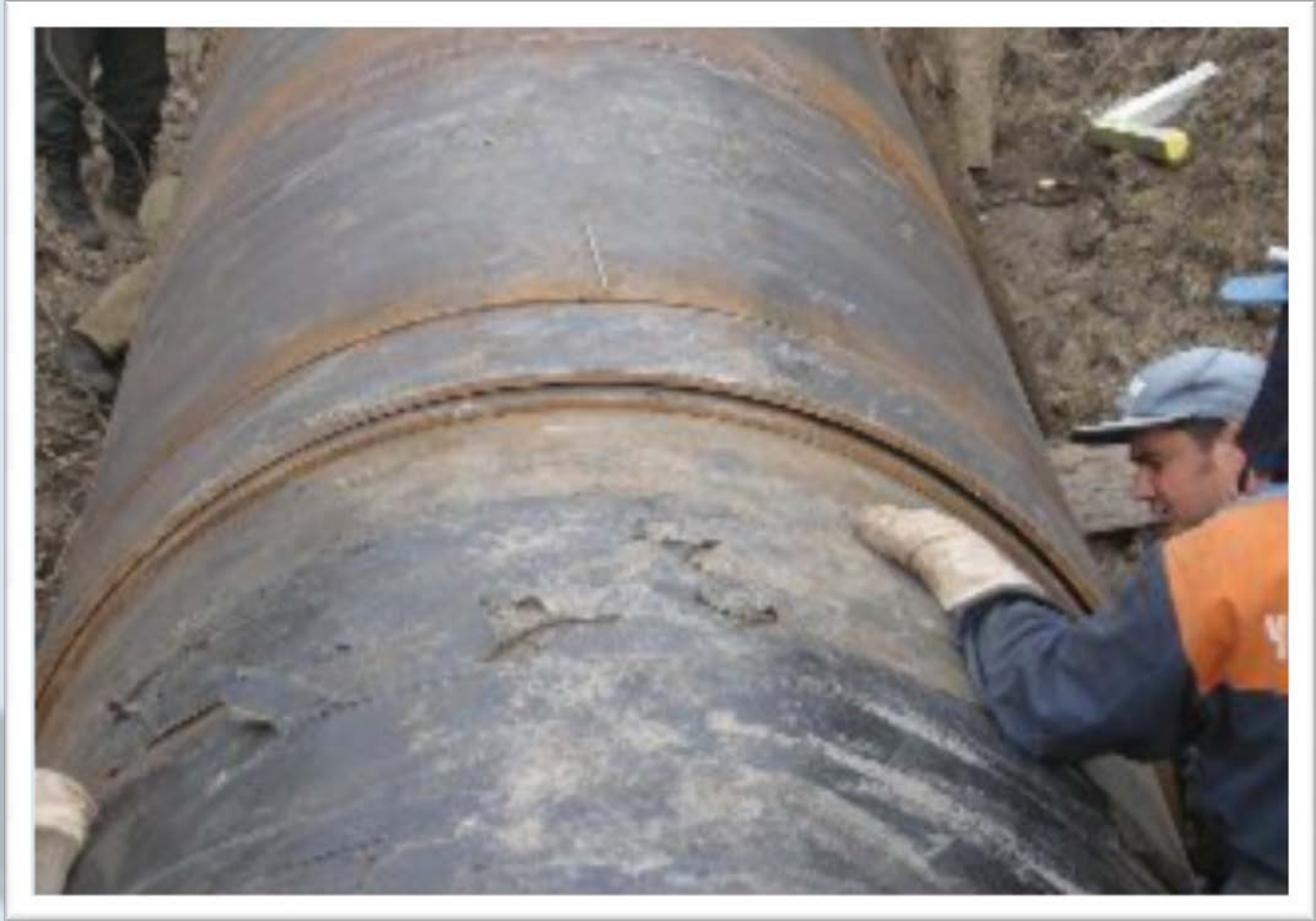
Figure 5: Application of two-layer sleeve
