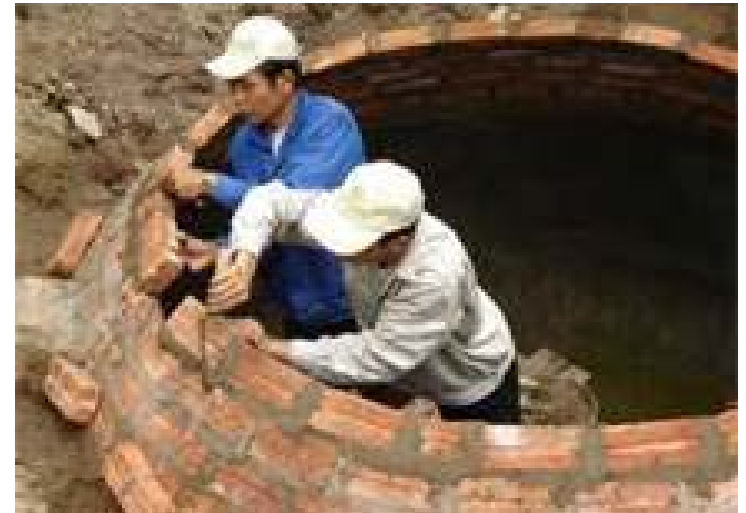
Fixed dome biodigester – SNV (For more information on SNV's Biogas Program: http://www.snvworld.org/ )
