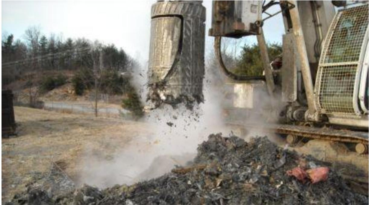
**Figure 3-5. Vertical Extraction Well Drilling**
