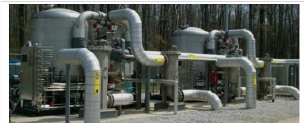
Figure 4-11. Siloxane removal systems at the Lorraine power station at Oberlin, Ohio, USA
