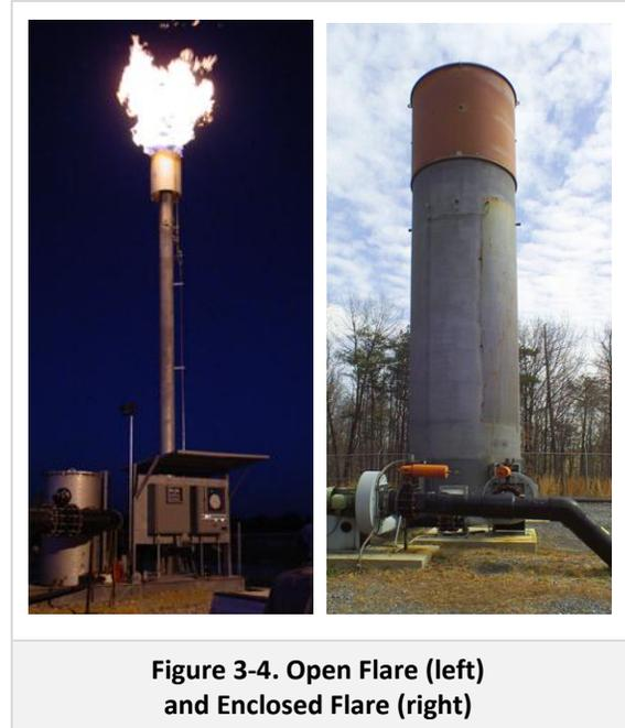
**Figure 3-4. Open Flare (left) and Enclosed Flare (right)**
