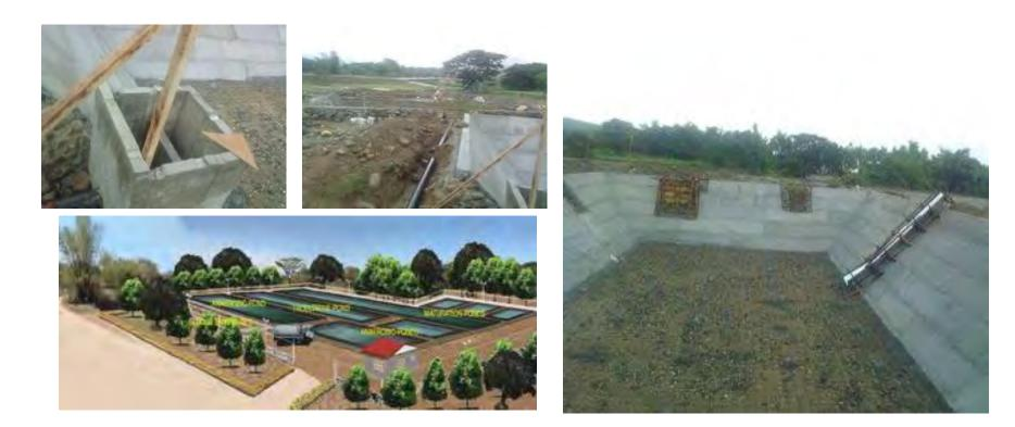
Septage management – Dumaguete City septage lagoons under construction, may add methane sequestration and capture system
