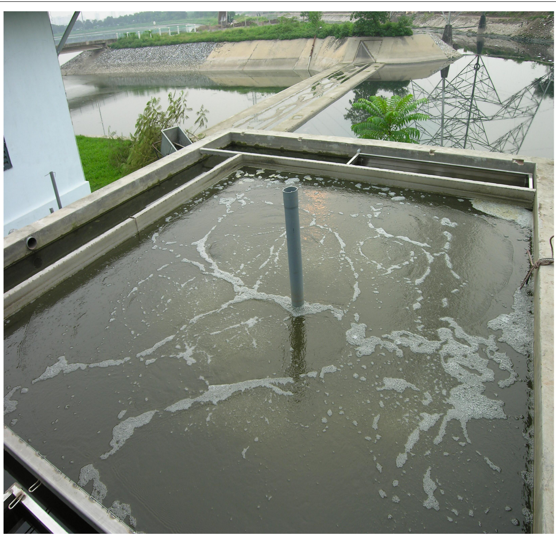
Treatment pilot plant of 93m 3 treated municipal wastewater from Kim-Nguu canal in Hanoi
