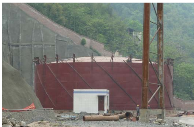
10,000 m 3 Gas Storage Tank, Yanjing Mine, China
