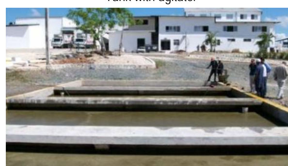
Sedimentation tanks
