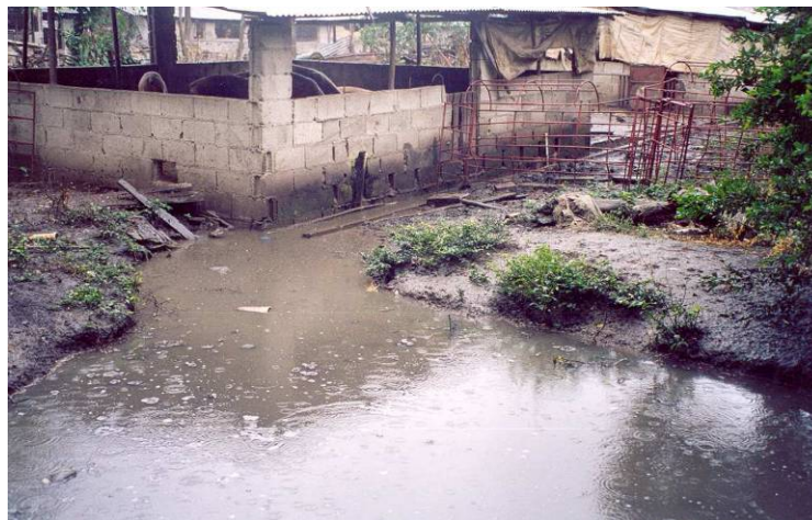
Figure 2.2 – The Open Anaerobic Lagoon Before the Project
