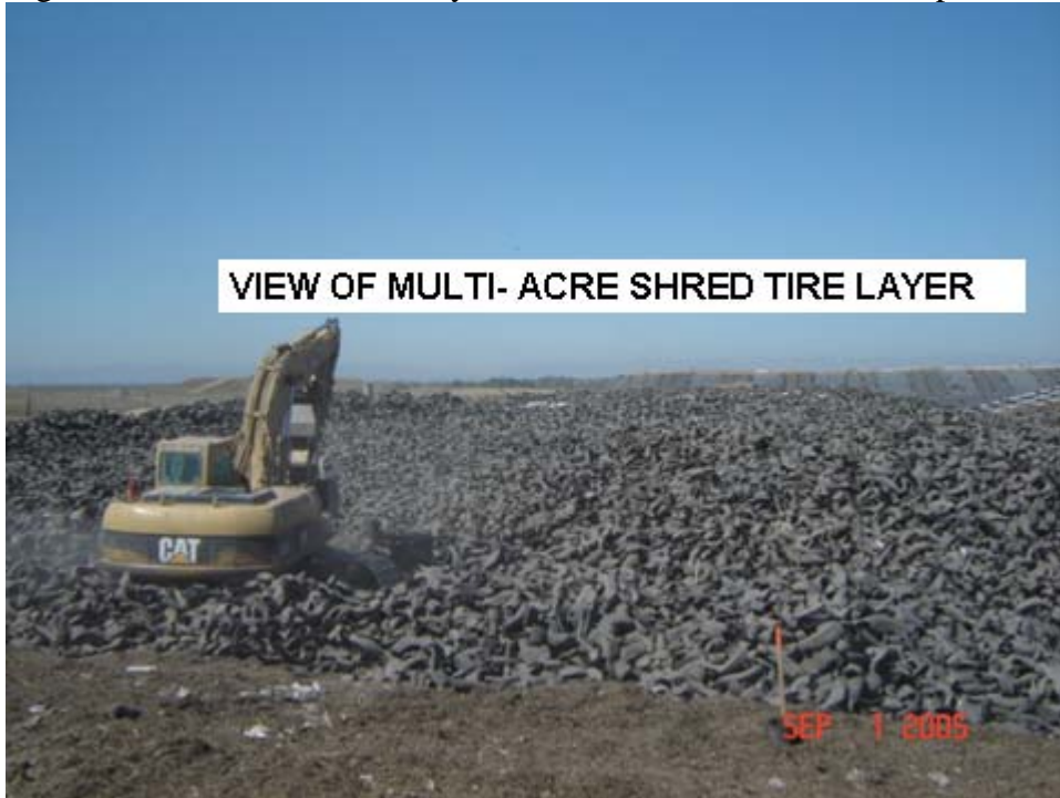
Figure 7. Photo of extensive layer of shred tires which will form permeable layer.
