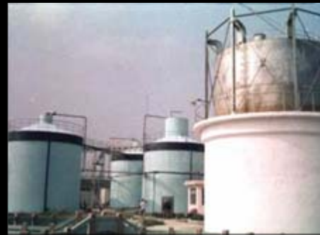
Project activity condition: Biogas digester with co- generation and aerobic treatment of liquid residue
