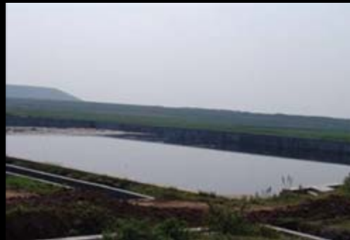
Pre-project activity condition : uncovered lagoon
