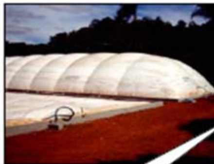
Project Activity Condition: Anaerobic Digester with Co-Gen and Flare
