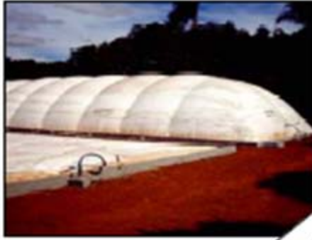
Project Activity Condition: Anaerobic Digester with Flare
