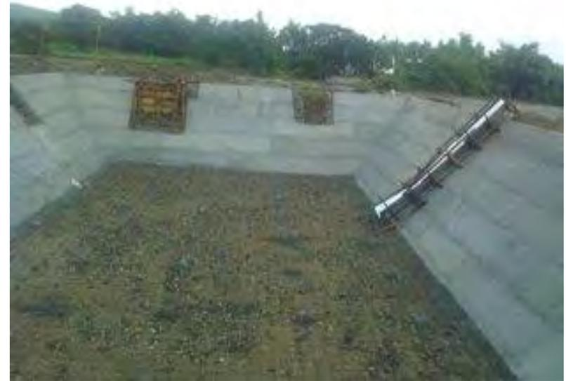
**Septage management – Dumaguete City septage lagoons under construction, may add methane sequestration and capture system**
