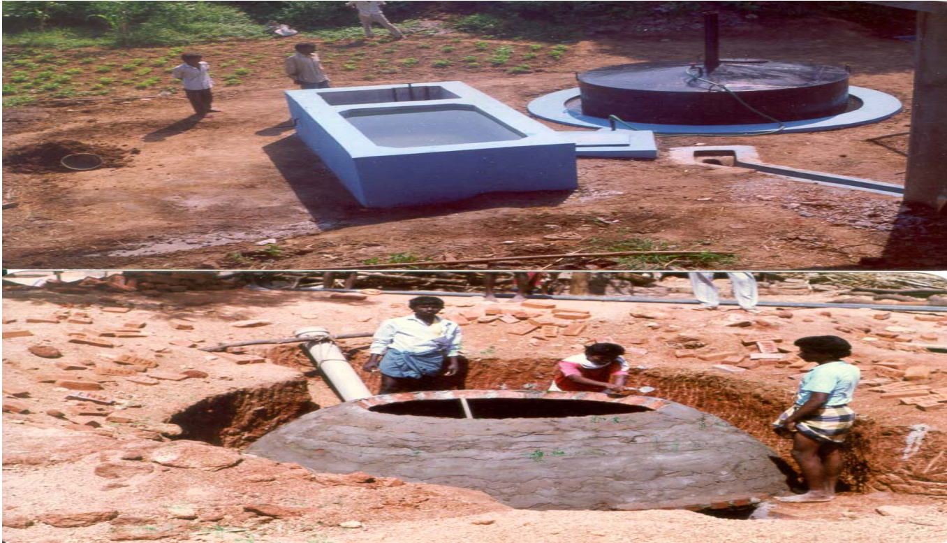
Biogas Plant Designs Top: Floating drum Bottom: Fixed dome
