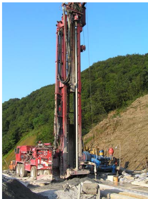
Surface Drilling Rig, Guizhou Province
