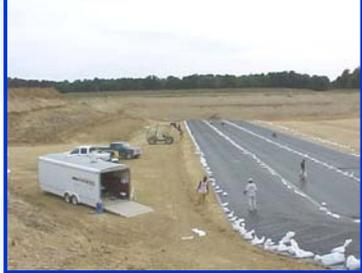
A 60 mil HDPE plastic liner is placed on top of the soil liner as the first phase of the leachate collection layer.
