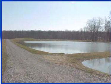
Rainwater that does not come in contact with trash is collected in sediment ponds.
