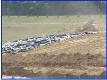
The working face is covered at the end of the day with a geo-textile tarp or 6 inches of soil to keep odors down and rodents away.
