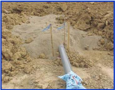
Perforated PVC pipe is then installed. This layer is the main leachate collection level and will collect liquids that seep through the trash.
