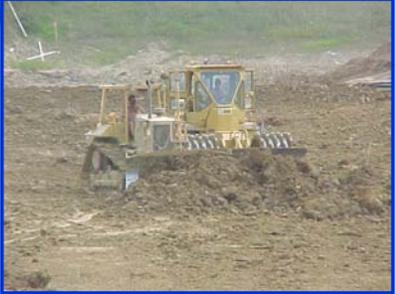
The leachate collection pipe and plastic liner are then covered with a protective layer of soil 18 inches thick.
