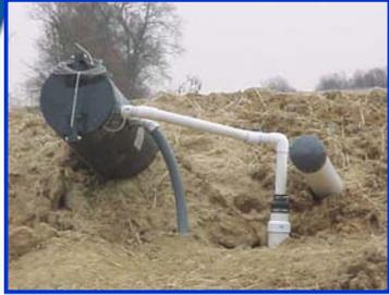
Collection pipe is installed to pump percolating fluids from the disposal cell to the leachate holding pond.
