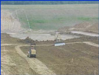
An 18 inch sand layer will contain perforated PVC pipe to collect leachate in case of main collection level failure.
