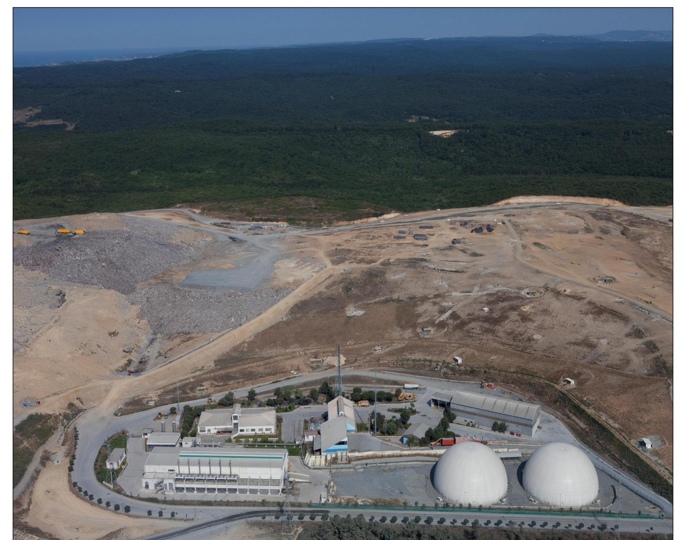
LFG Energy Plant
