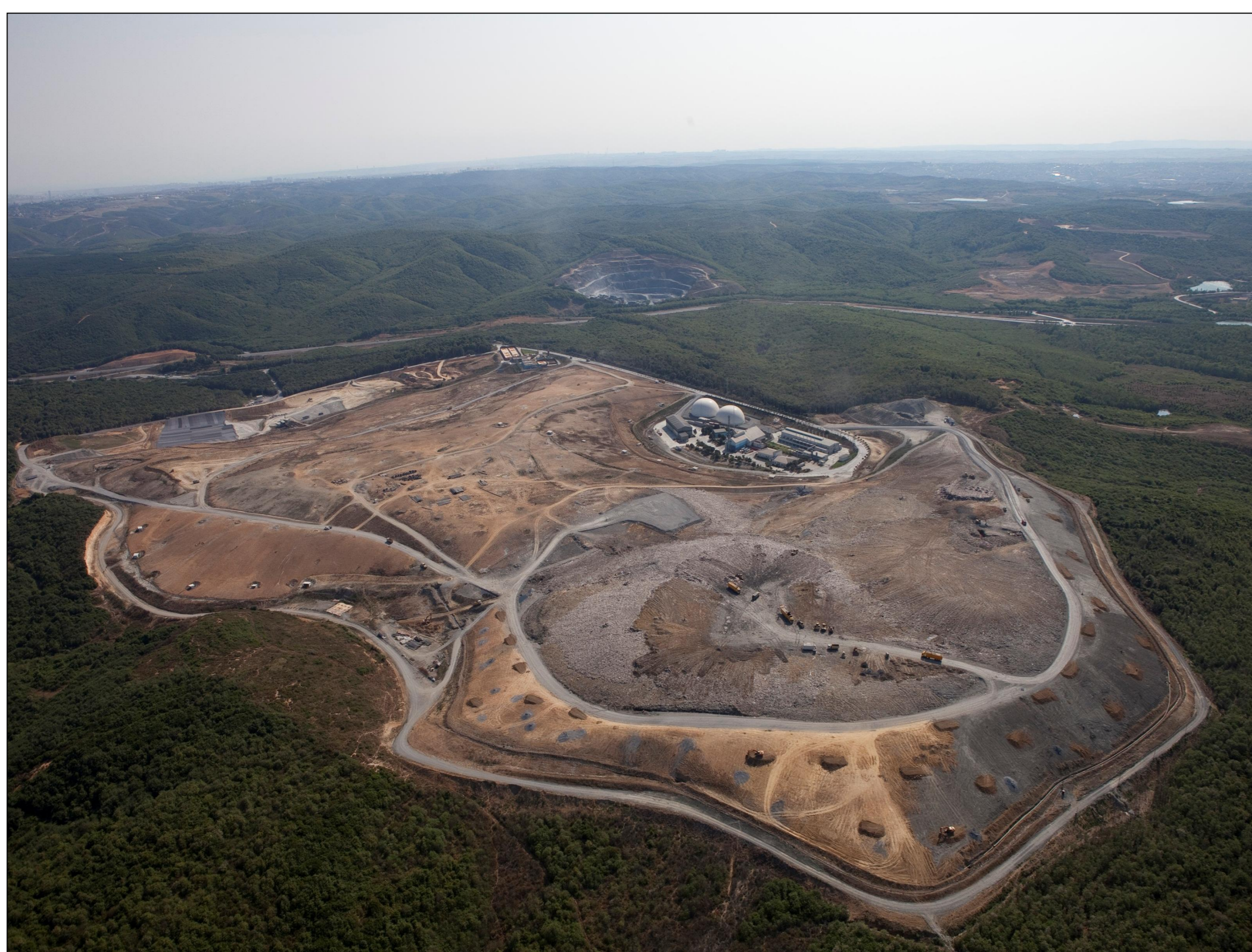
Aerial View of Landfill
