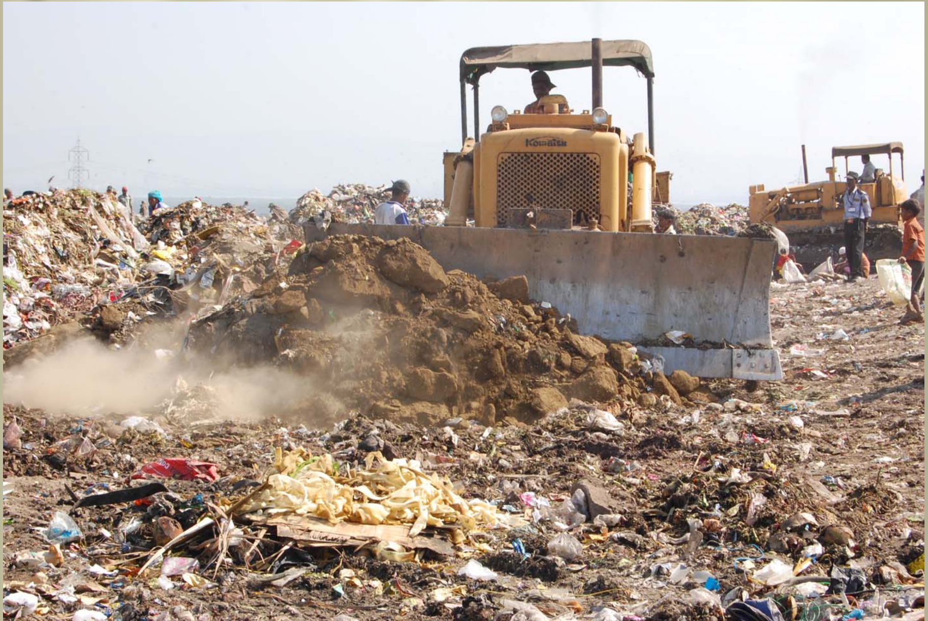
TOP SOIL COVERING OVER FRESH MSW AT LOOP NO - 8
