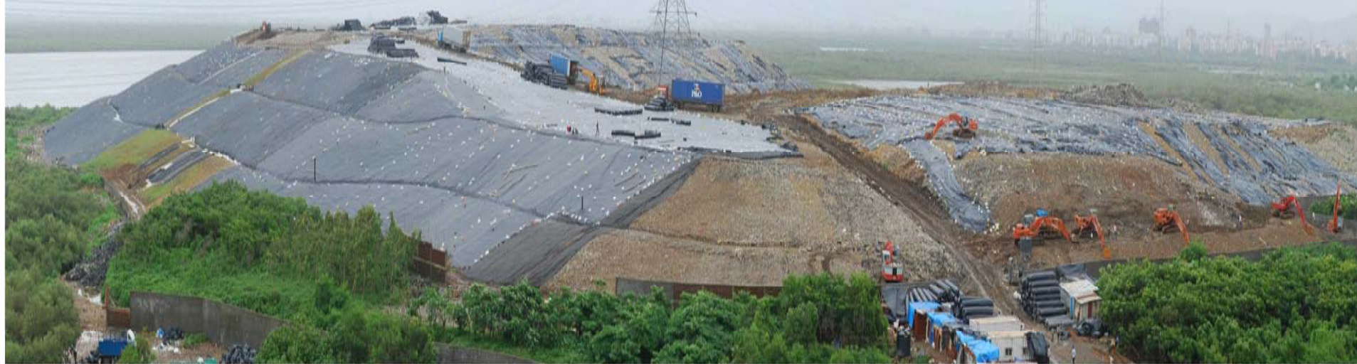
PROJECT : GORAI DUMPING GROUND AS ON AUG. 2008
