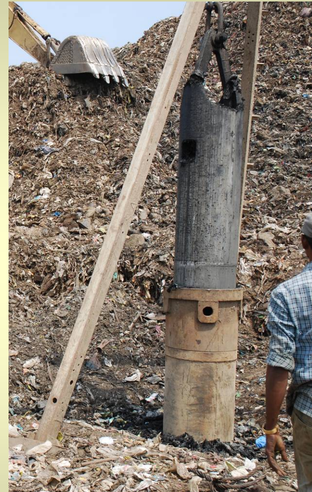
Construction Procedure followed at one of our sites
