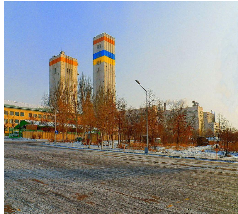
The main building of PJSC “DTEK Mine Komsomolets Donbassa”*
