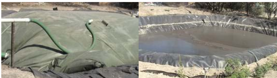
Figure 2.1 – Las Palmas Bag-Type Digester (left), Effluent Lagoon (right)
