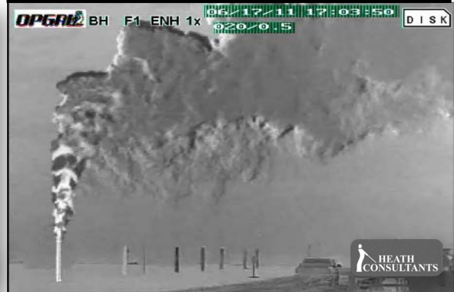
Compressor Station Blow Down Enhanced Mode
