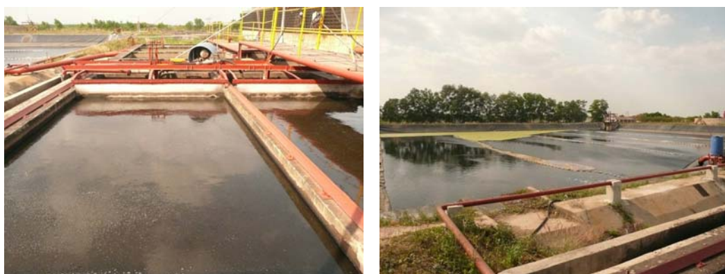
Figure 3.6 – The Wastewater Treatment System at Bourbon Tay Ninh
