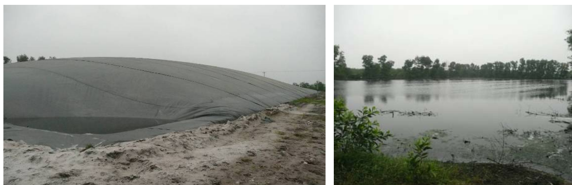
Figure 3.9 – The Covered Lagoon and One of the Seven Open Lagoons at Thua Thien Hue Cassava Factory
