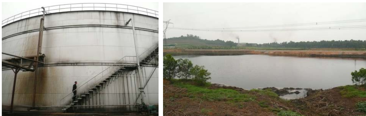
Figure 3.7 – SMAG Reactor and Open Lagoon to Treat the Wastewater from Ethanol Production at LASUCO
